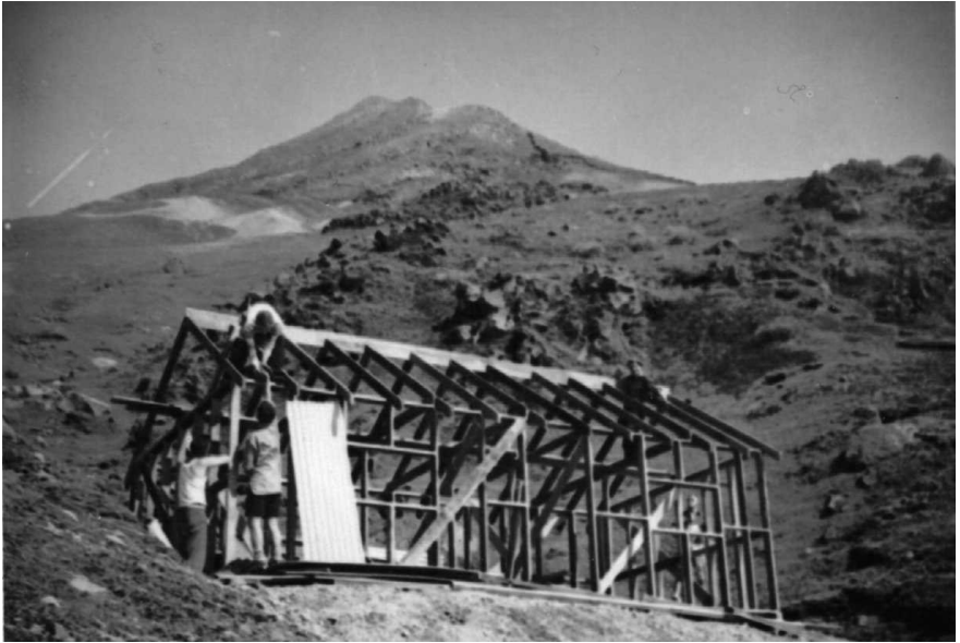
Starting Construction on Tahurangi Hut. — Dave Rawson collection
